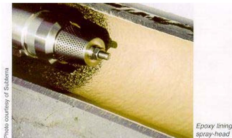
Various resin formulations are available, including high-build, thixotropic materials that resist sagging. Some water utilities have a preferred material or an approved list of materials for particular applications, and details will be included in the contract specification.
