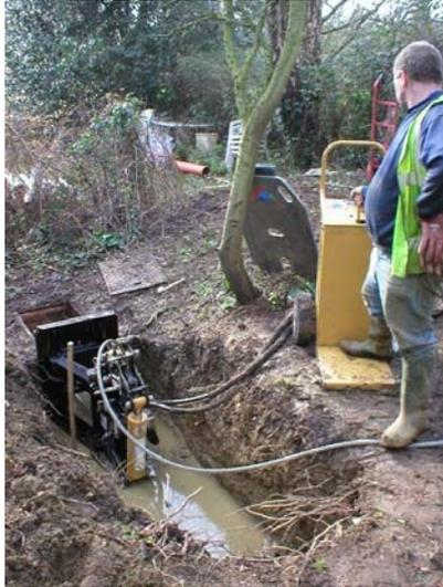
*A small footprint pipe bursting unit. Picture courtesy of Earth Tool Inc/U Mole Ltd*
