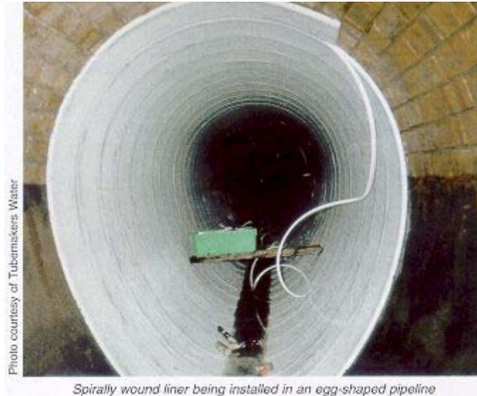
Other systems have interlocking profile edges rather than a separate locking strip, and one variant uses a self-powered winding machine, similar in concept to that used for spirally wound non-man-entry liners, which travels through the host pipe as it forms the liner. The system can create non-circular liners, the shape being determined by the configuration of the winding cage.
