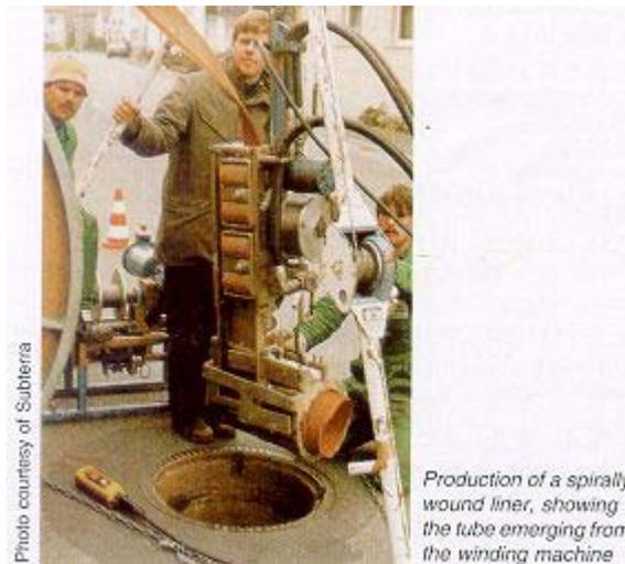
An alternative spirally wound technique uses a winding machine that travels through the host pipe as it creates the tube, thereby removing the need to rotate the liner itself. By using a winding cage shaped to suit the host pipe, non-circular sections can be lined, including ovoid, egg-shaped and rectangular.
