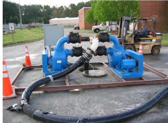
*A typical large-capacity bypass pumping system working from an existing manhole. Picture courtesy of Hampton Roads Sanitation District, Virginia, USA.*
