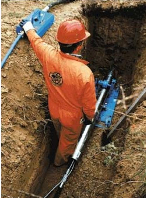
*Impact Moling hammer in its launch pit. Picture courtesy of Tracto-Technik.*
