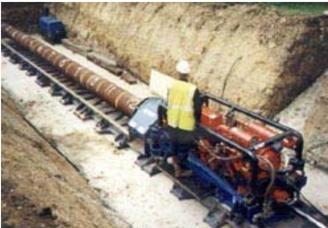
A Typical Auger Boring set-up. Picture courtesy of Allen Watson Ltd.
