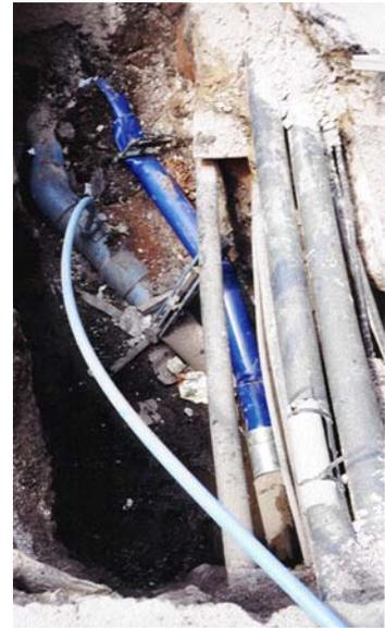
fig 2 close proximity of utilities in an access pit
