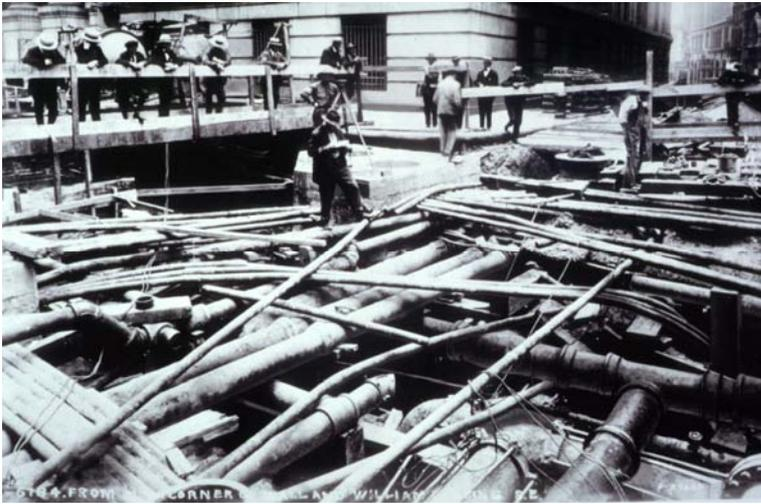
Fig 1 complexity of utilities just beneath a city street
