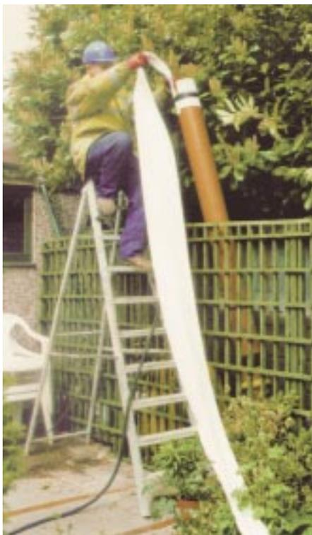
*Installation of an ambient-cure liner in a site with difficult access*
