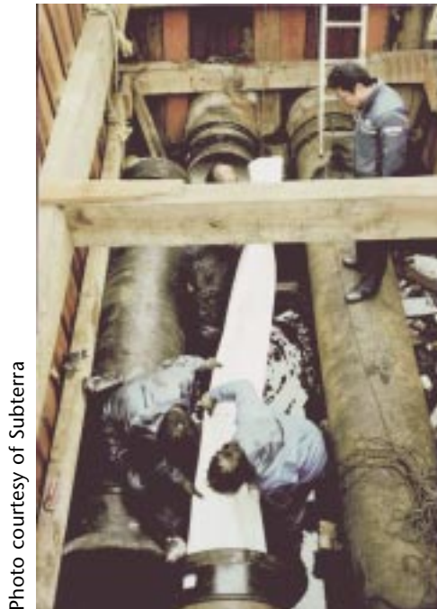
Localised repair using a short length of resin-impregnated liner tube
