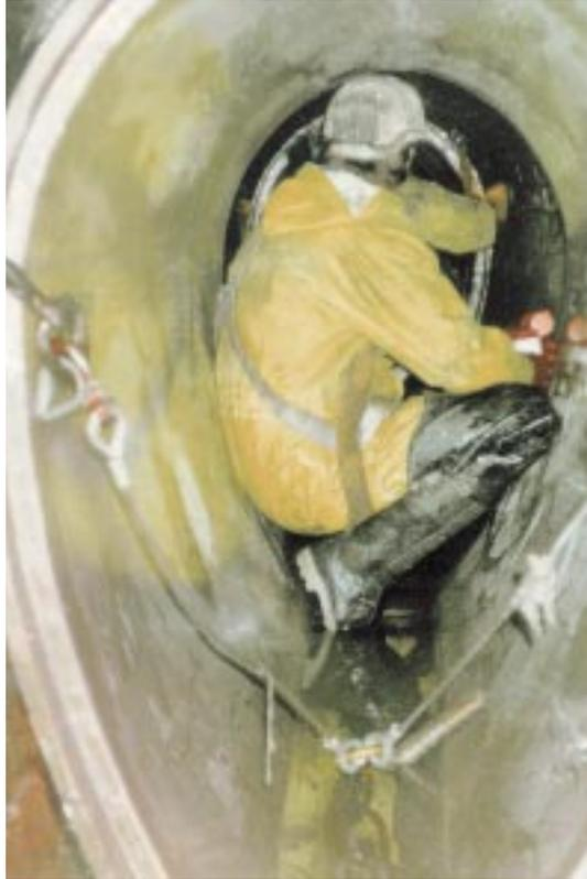
*Installation of GRP liner sections in a man-entry sewer*
