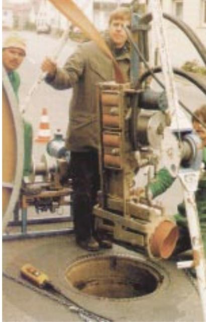
*Production of a spirally wound liner, showing the tube emerging from the winding machine*
