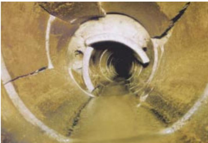
*Partial collapse of a clayware sewer, revealed by CCTV inspection*
